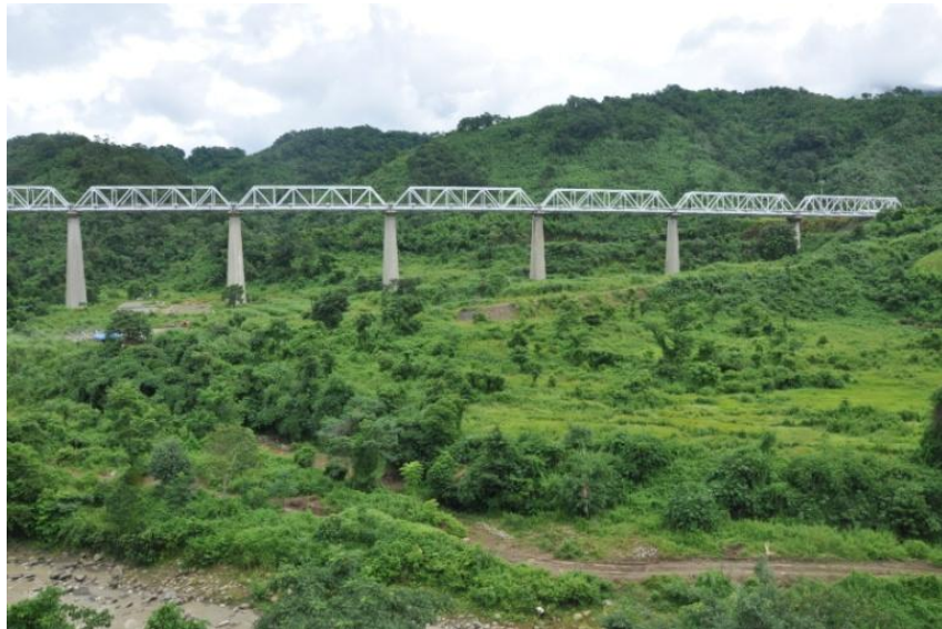
Newly completed Dayang Bridge near New Haflong Station
